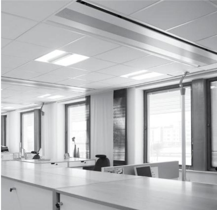
**Figure 36: Krueger Chilled Beam Office Application.**
