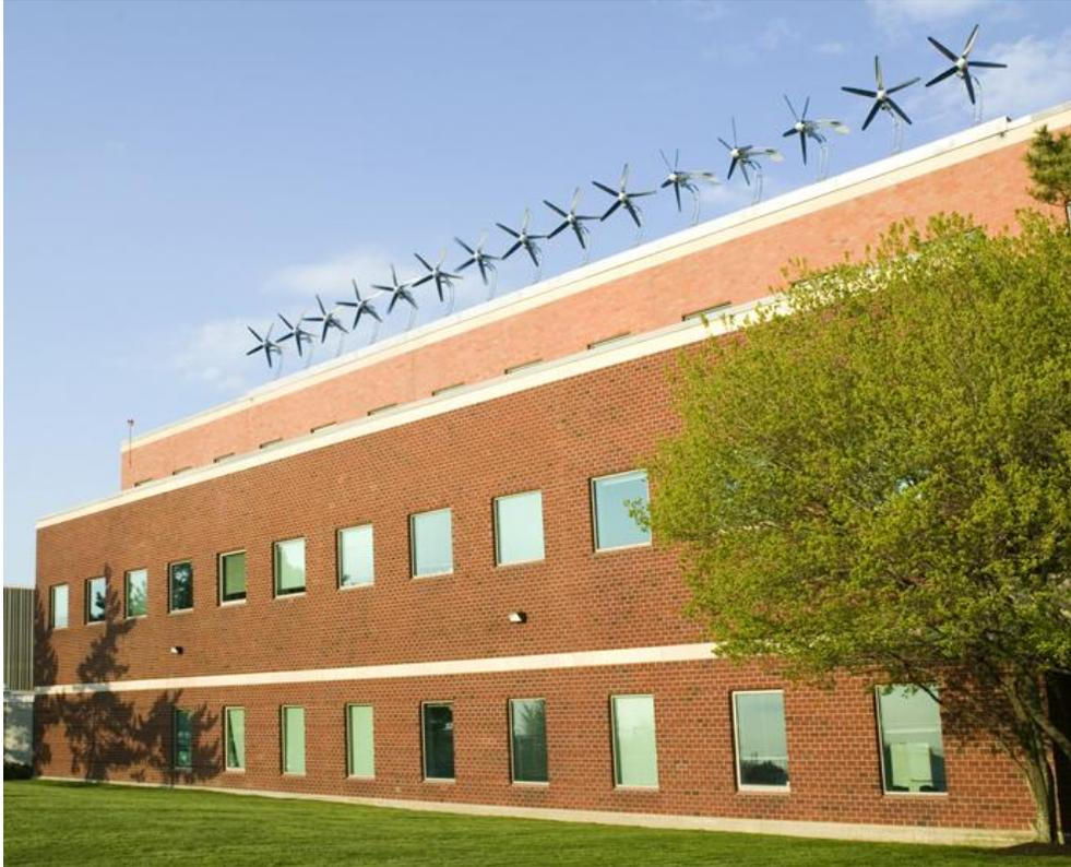
**Figure 183: AeroVironment Architectural Wind Building Integration.**
